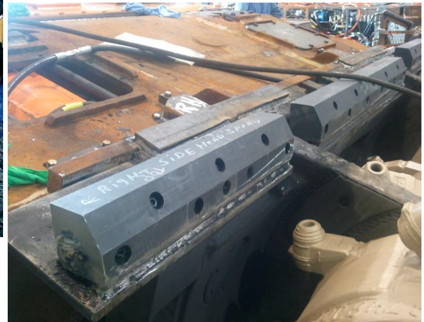
Installation of sprays at JOY rebuild center – SLD sprays
